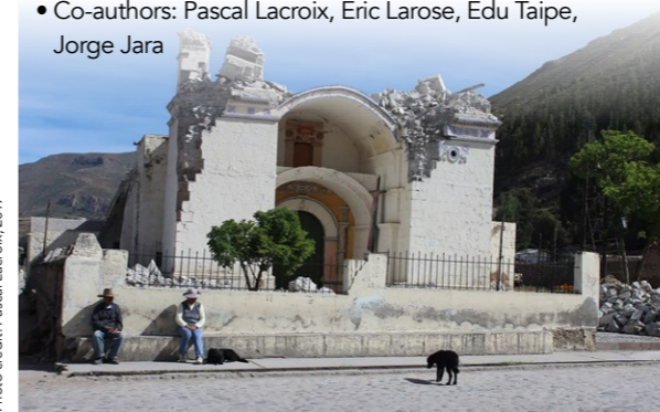
Ichupampa church, just 10km from Maca, was destroyed by a magnitude 5.5 earthquake in 2016.
