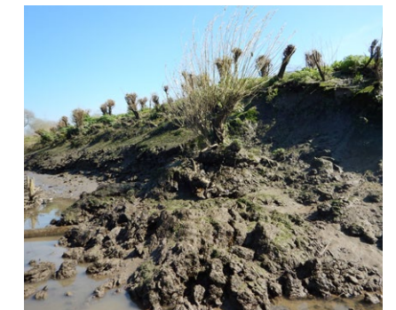
Liquefaction of the river bank with descending willow in the middle.
